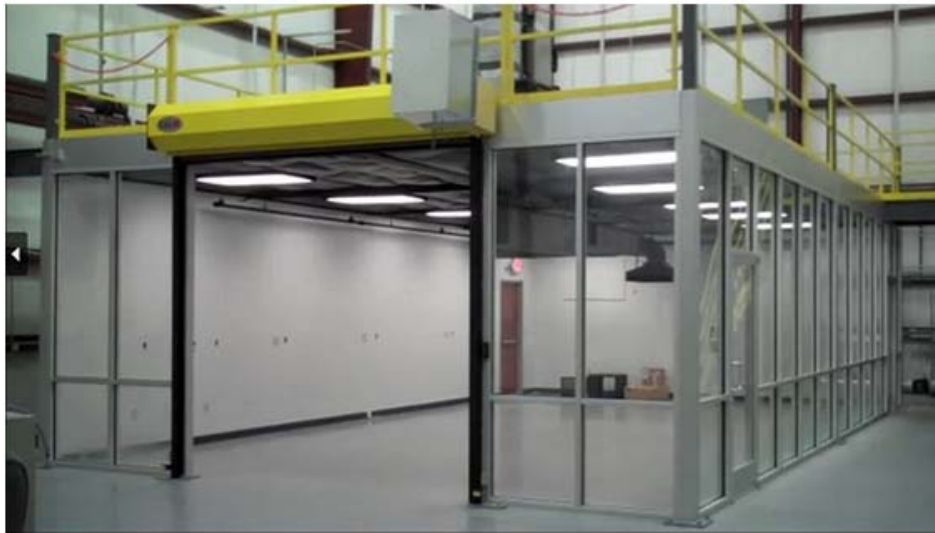
Our new lab facility structure is complete
